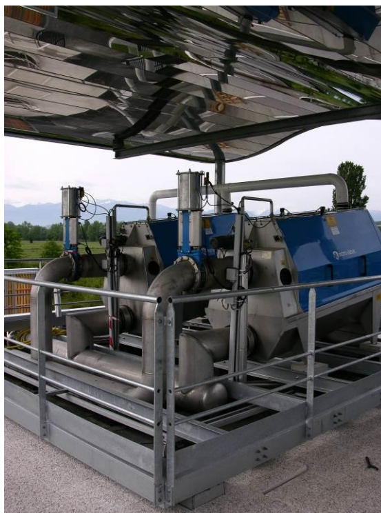
Illustration 11 : Tamis Step Assat-Bordes
